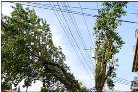
Directional pruning in proximity to a circuit body.
